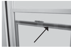
Check rail weatherstrip - Exterior view
