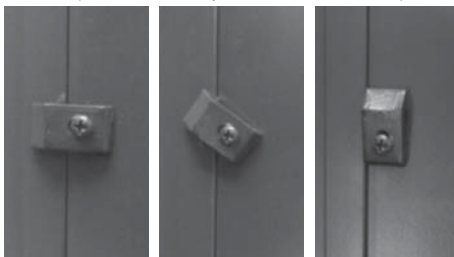
Secured position Partially unsecured Unsecured position
