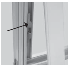
Lock mechanism - Exterior view
